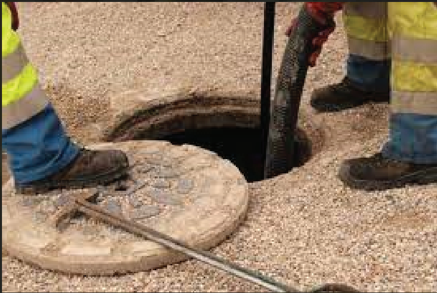
Cleaning of underground chemical storage tank (Shell and tube)
